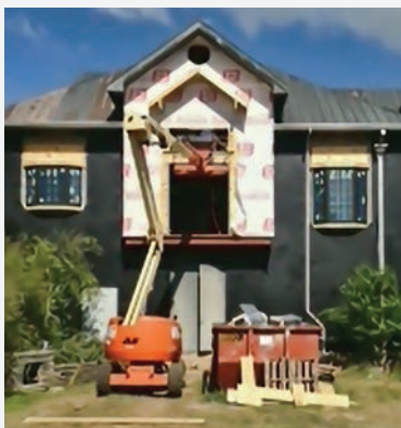
External view of construction
